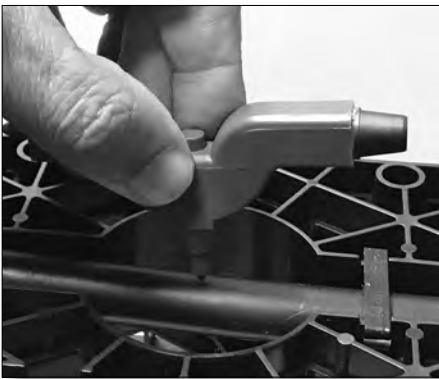
4. Puncture the poly pipe with a 4mm punch tool.
