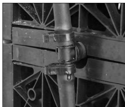
8. When all Drip Emitter are installed, rotate the poly pipe 90 degrees.
